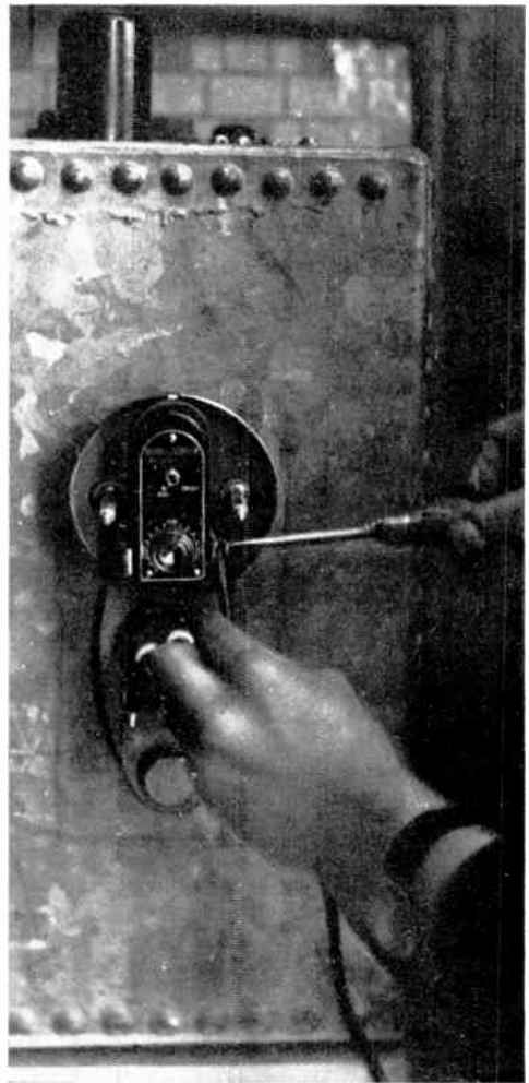
Fig. 8.—WIRING CONNECTIONS BEING MADE TO THERMOSTAT.
