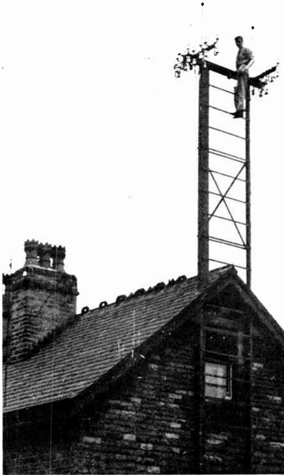
Fig. 1.—RADIO RELAY STATION DISTRIBUTION MAST. (By courtesy of J. S. Ramsbottom & Co., Ltd., Bow Street, Keighley.)
