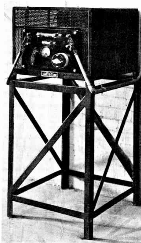
Fig. 3.—WESTINGHOUSE 500-WATT COPPER-OXIDE RECTIFIER FOR TRICKLE CHARGING THE BATTERY ILLUSTRATED IN FIG. 4. (Courtesy of The Westinghouse Brake and Saxby Signal Co.)
