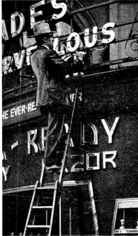
FITTING UP A NEON TUBE ON A SIGN AT FACIA HEIGHT.
