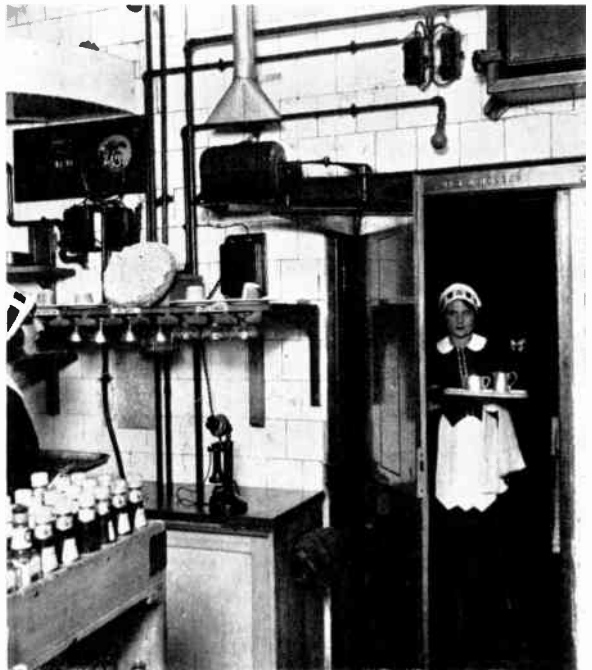
THE MECHANISM WHICH CAUSES THE DOOR TO OPEN. Showing the arrangement of the actuating mechanism.
