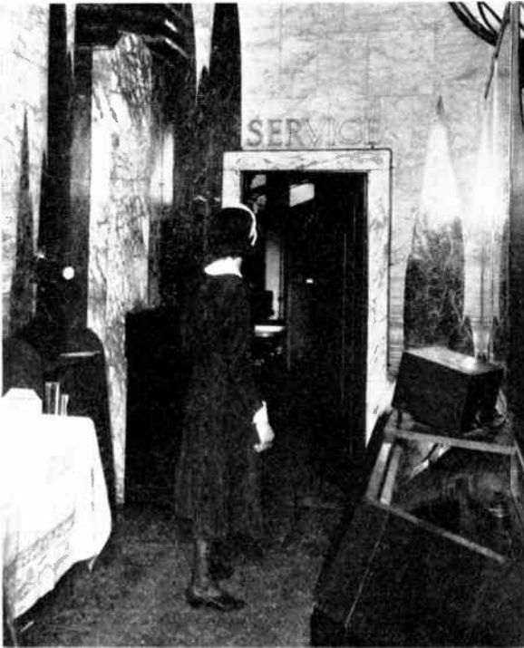
THE SELF-OPENING DOOR AT THE "OXFORD" CORNER HOUSE.
