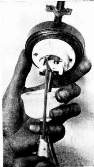
FIXING CEILING ROSE TO BLOCK AND MAKING CONNECTIONS.
