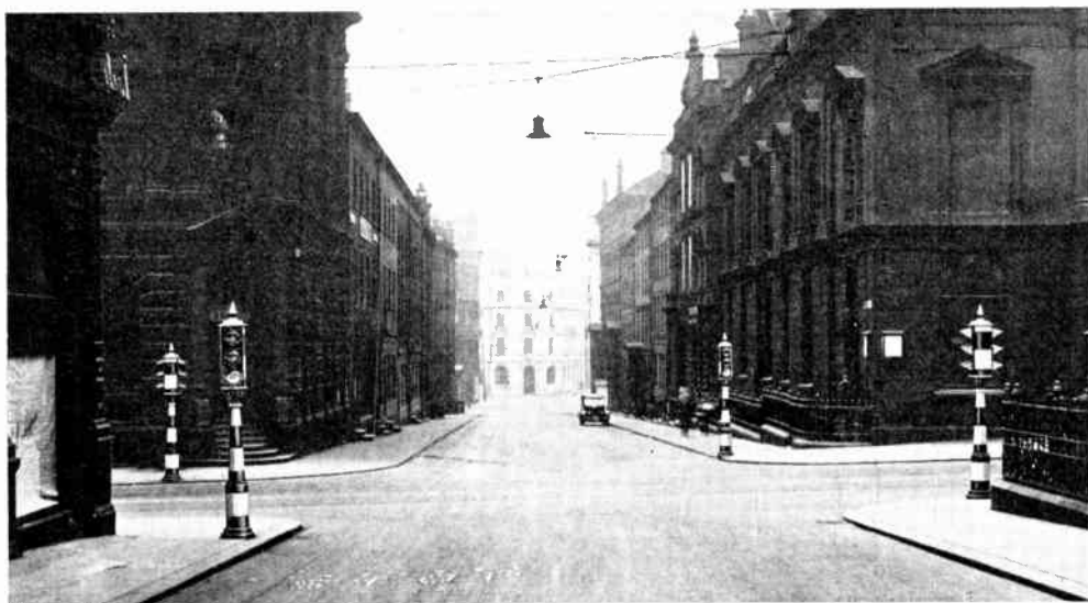
A TYPICAL TRAFFIC SIGNAL INSTALLATION. This shows four two-way traffic signals in operation.
