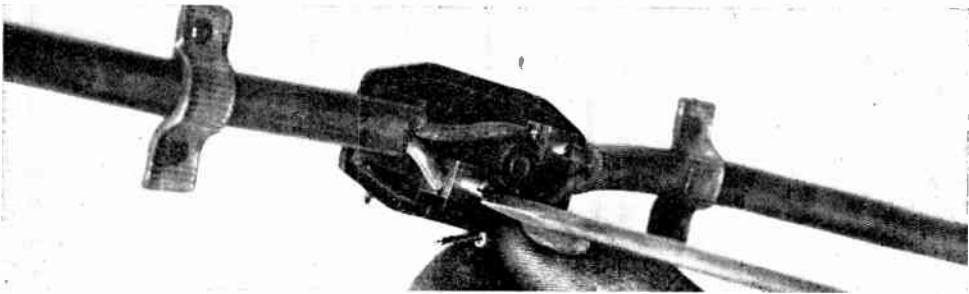
HOW TO MAKE A JOINT, USING THE STANDARD C.R. STRAIGHT-THROUGH (TWO-WAY) CONNECTOR BOX.
