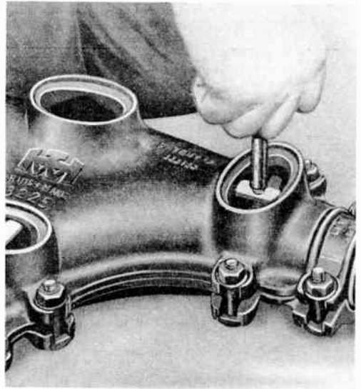
TIGHTENING THE SHUTTLES ON TO LEAD BONDING STRIP.
