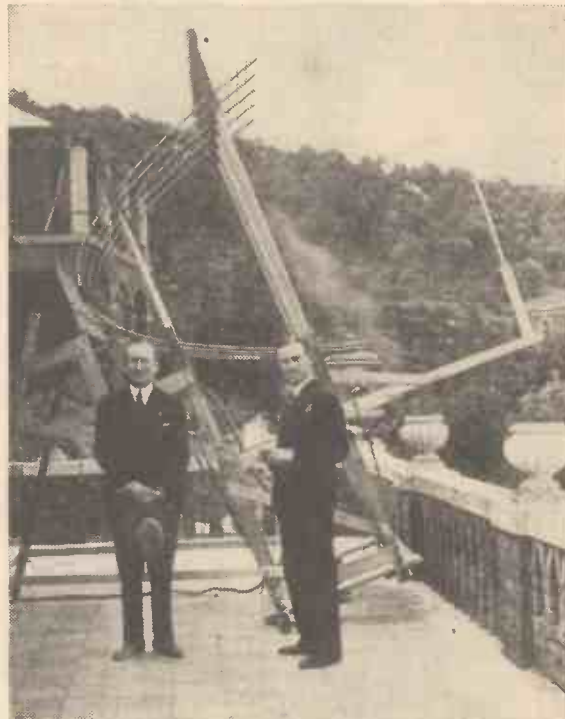
Courtesy, Marconi's Wireless Tel. Co. The great inventor standing beside his experimental 57-centimetre ultra-short-wave aerial erected at the Rocca di Pana, near Rome. With this equipment messages were sent to Cape Figari, Sardinia, a distance of 168 miles.
