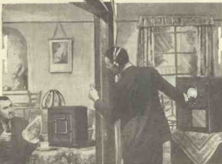
For the first try-out of the set it is a good idea to arrange the speaker and the receiver near to a door but on opposite sides, as illustrated by this photograph. It is then an easy matter for the listeners on both sides to compare notes.
