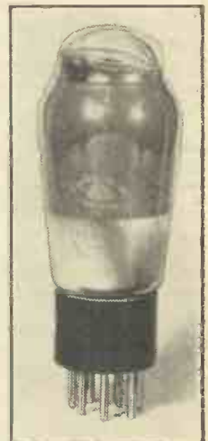
The new Mullard Pen. 4VB, a steep-slope output A.C. pentode.
