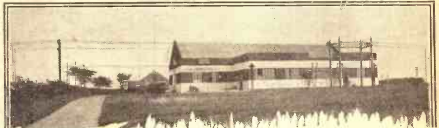
The station building of the Empire broadcasting service photographed shortly after its completion. In a few months the Empire short-wave service, which cost about £40,000 to start, will celebrate its second birthday.
