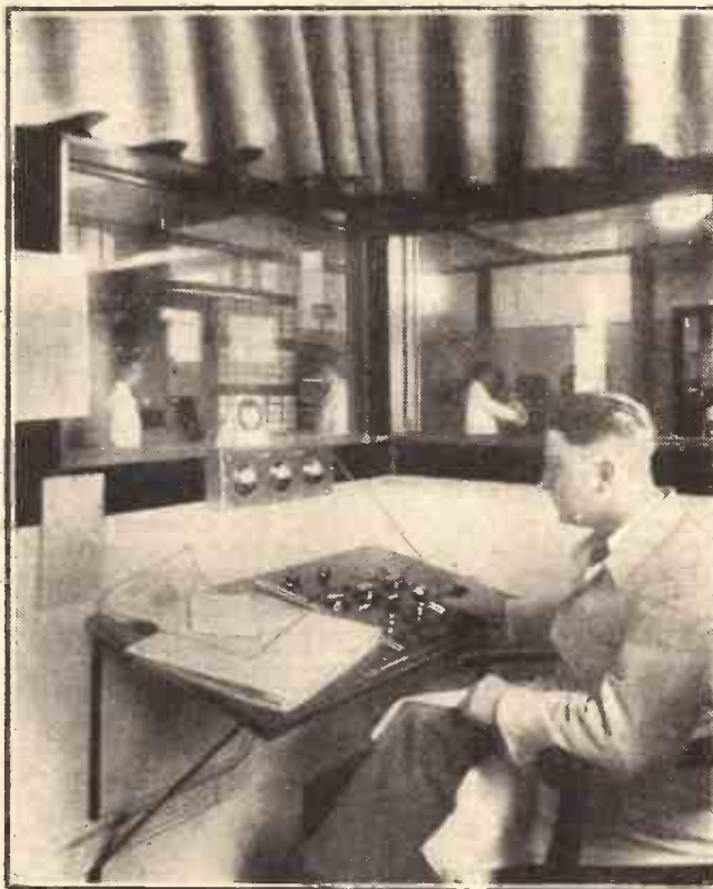
The main control-room or "inner sanctum" of the engineers' department in Broadcasting House, Berlin. From this small cabinet the man in charge can keep an ear on the programmes and an eye on the rest of the department.
