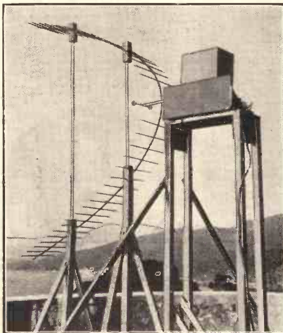
No, it's not part of a switchback railway or children's slide, but the curious beam aerial used for getting down to the shortest of short waves. The actual installation to which this aerial belongs works on a wavelength of 16 centimetres!
