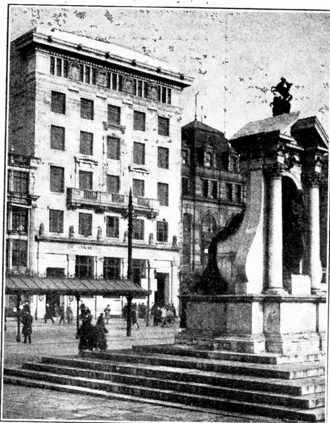
A view of Broadcasting House, Manchester, which is, at the moment anyway, the most complete and most modern broadcasting centre in Britain
