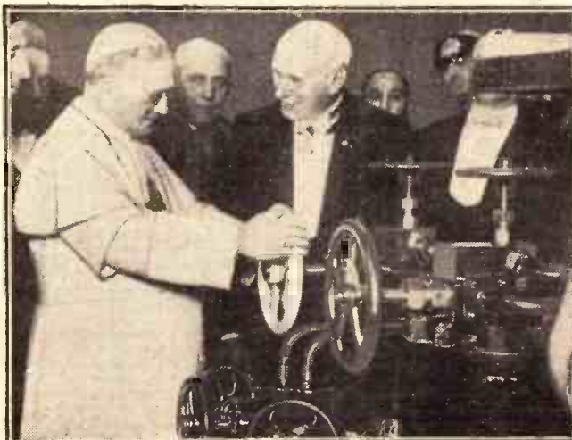
Pope Pius XI opens the electric power station which now supplies the Vatican City with current for lighting and heating and for the radio installation.
