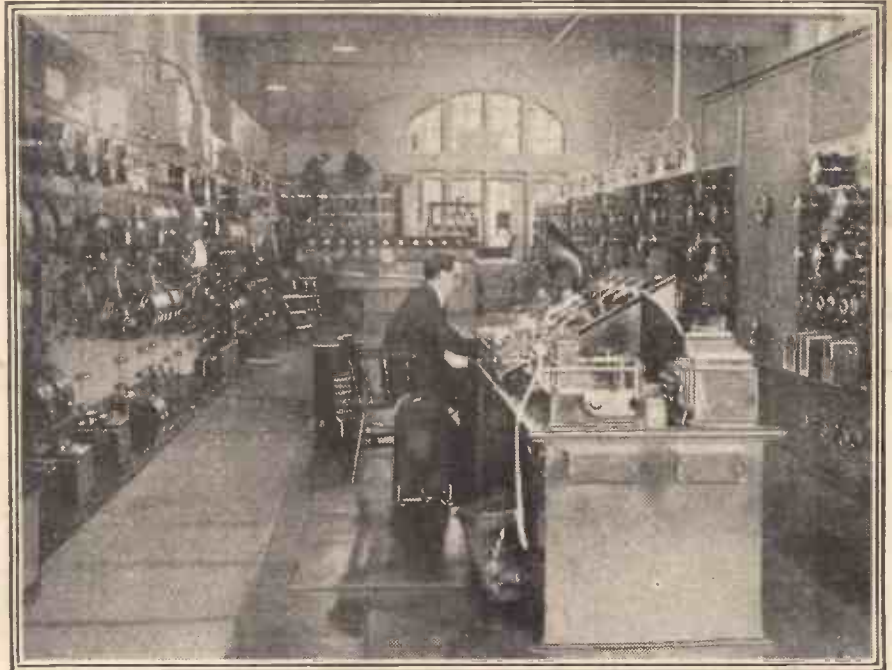
A great deal of the control of Königswusterhausen is carried out in the switch-room shown above where the power control plant is situated.
