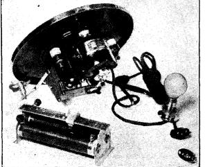
An electric gramophone-motor complete with control rheostat.
