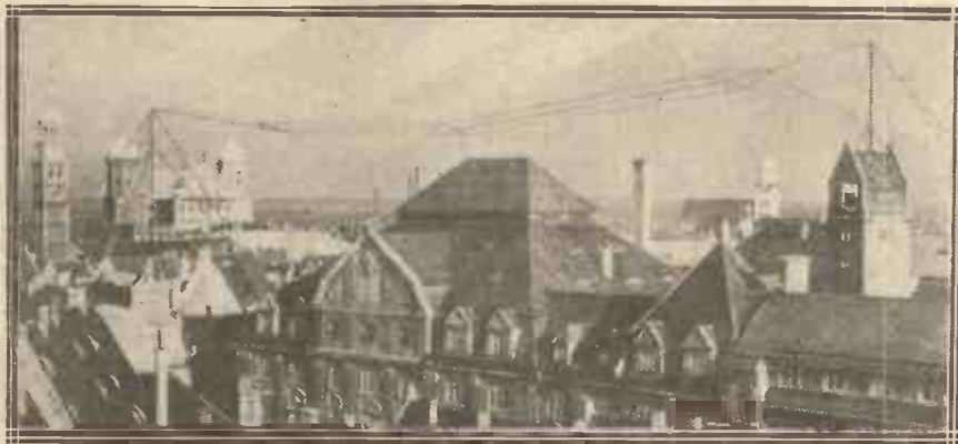
The aerial of Augsburg, one of the German relay stations that transmit the Munich programmes. Its wave-length is 560 metres.
