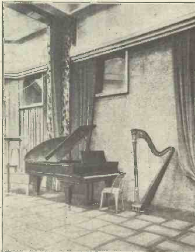
A corner of the great new studio which has been built at the Radio-Paris broadcasting station. Adjustable velvet draperies are provided to govern the studio's acoustical properties.
