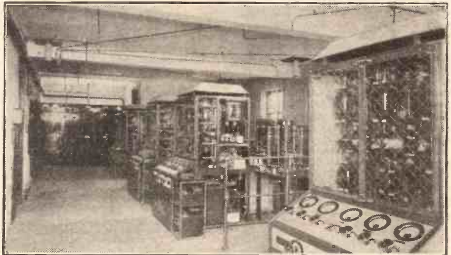
The main radio transmitting-room at London's Air Port, Croydon. There are four Marconi 3 kw. transmitters, which can handle C.W., "Tonic Train," or Telephony on any wave-length between 800 and 2,000 metres.
