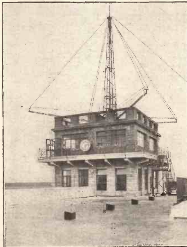
The new control tower at the Croydon air port. This photo is taken from the roof of the main building, and clearly shows the Marconi D.F. aerials suspended from the 54-ft. centre mast.
