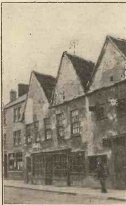
A cage type of wireless aerial is to be seen above one of the oldest buildings in Ross-on-Wye, Herefordshire.
