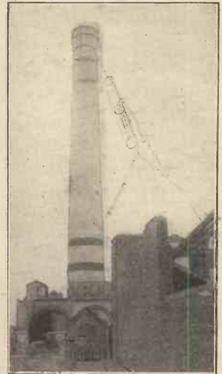
5 W A's aerial is suspended from the Power Station chimney.
