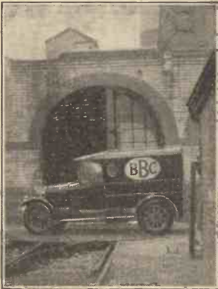
The entrance to the building which houses 5 W A's transmitter.
