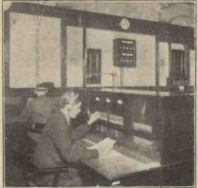
The London switchboard and indicator for simultaneous broadcasting.
