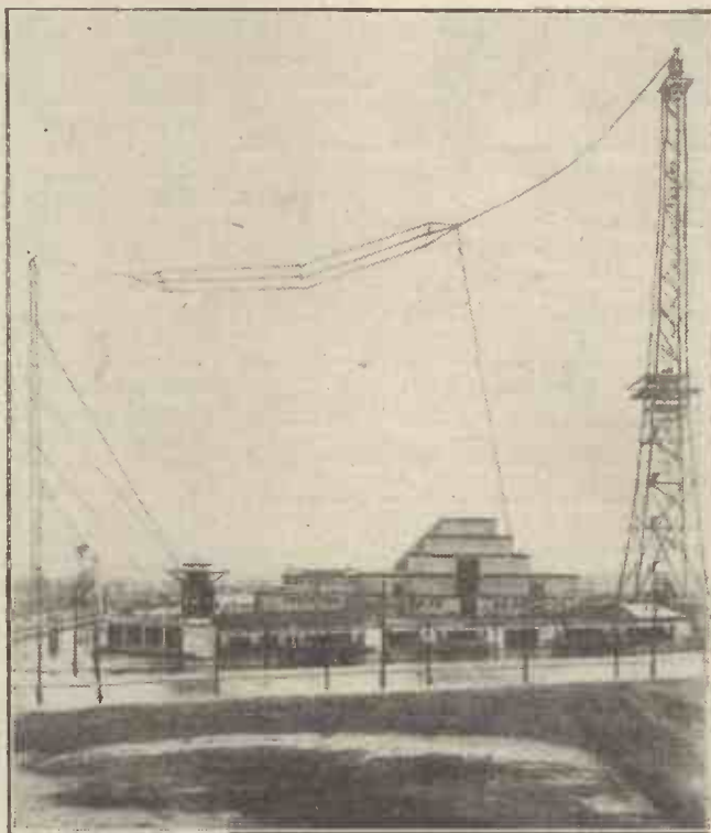
Aerial system of the Witzleben broadcasting station. This is situated near Berlin.
