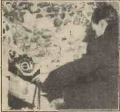
Fixing the microphone in a church tower, for broadcasting the bells.
