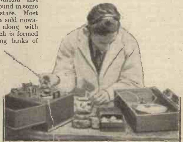
Fig. 6. Testing samples of radio crystal before placing them on the marks.
