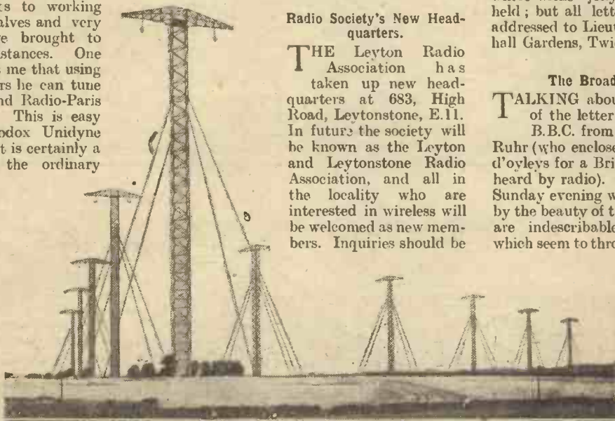
The new Bridgewater Beam Station. On the left are the five masts for receiving from Montreal. The other five masts (to the right) will support the aerial that listens for South Africa.
