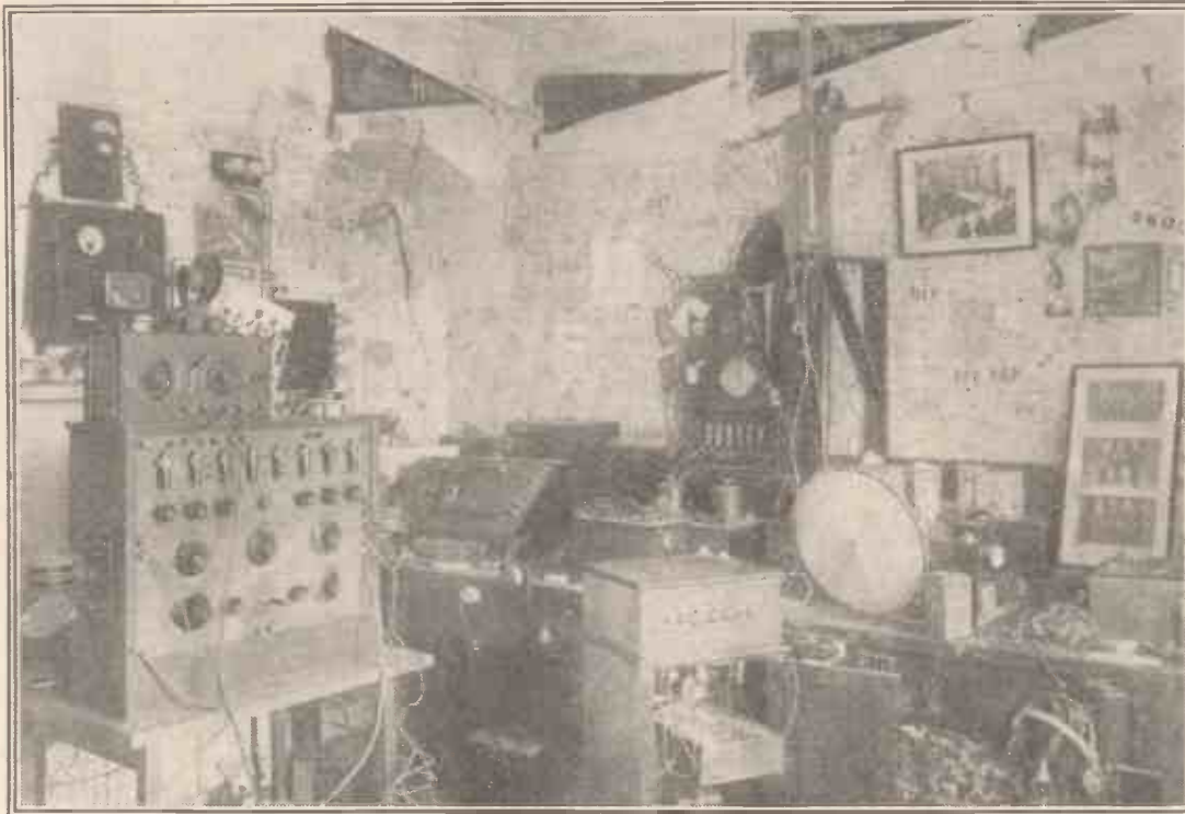
The general receiving and experimental room at 2 N M. The set on the left is an 8-valve super-heterodyne.
