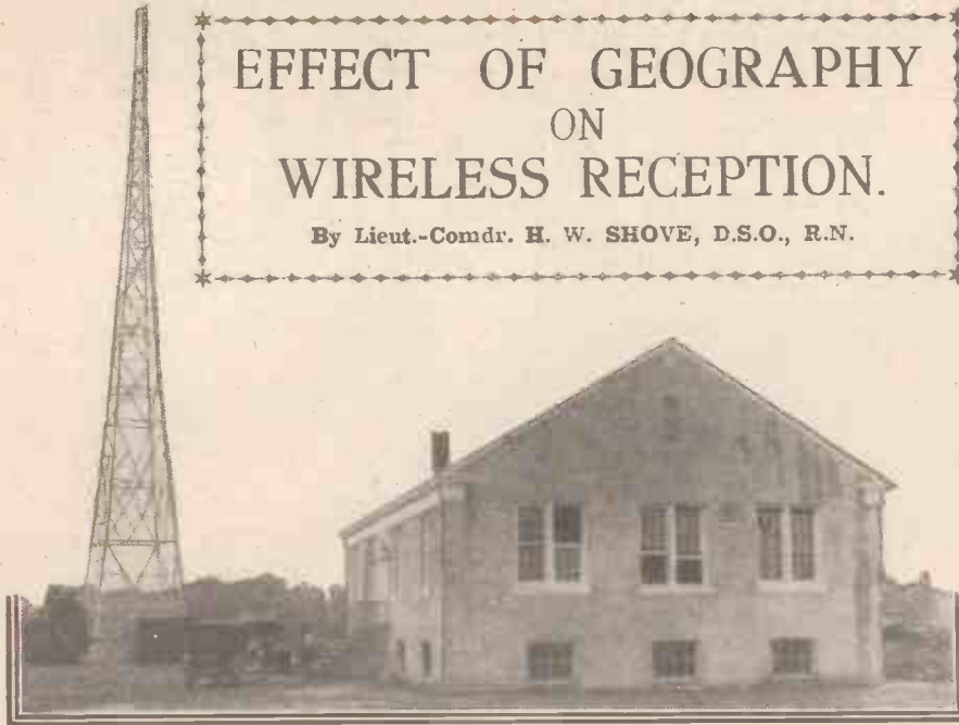
One of the masts of the nearly completed 50 kw. broadcasting station (W J Z) at Bound Brook, New Jersey.
