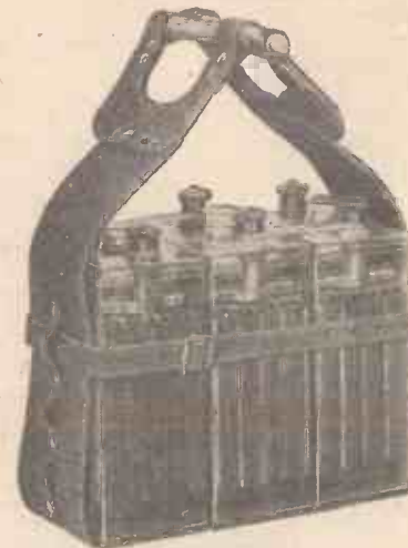
Carrying 6 Volts 40 Amps.
