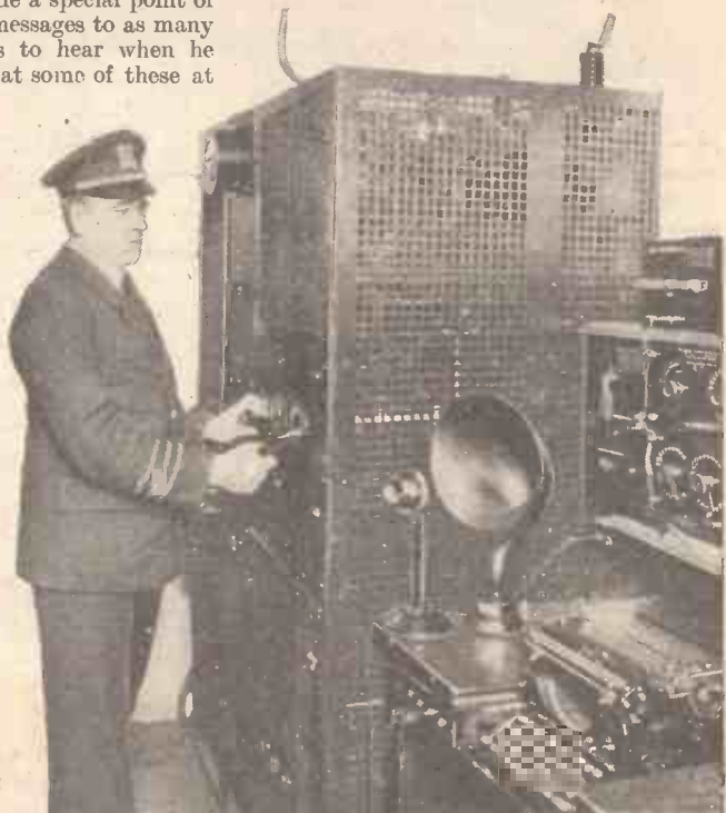
The chief operator of the "Leviathan" adjusting the C.W. transmitter.
