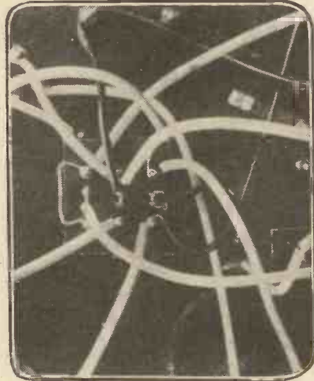
Fig. 9. A "close up" of the wiring of the switch.
