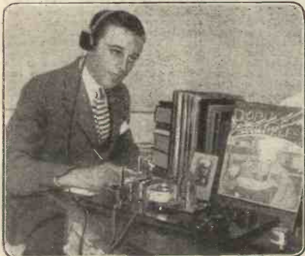
POPULAR WIRELESS is known pretty well all over the world by now. Here is a photograph sent in by a reader in Malta, showing an automatic Morse machine used for speed tests.
