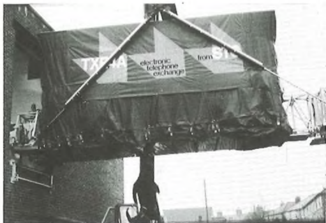
FIG. 2—Largest module being manoeuvred by telehoist
