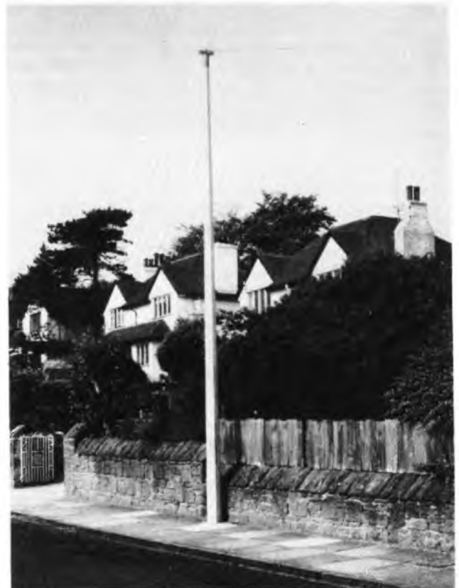
FIG. 1—The hollow pole
