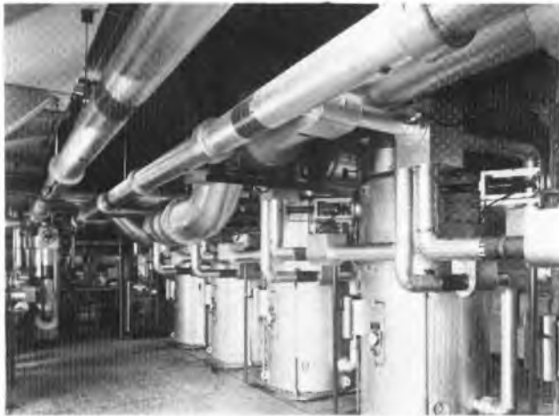
FIG. 9—Waste-heat boilers
