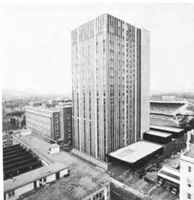
FIG. 1—Cardiff telephone exchange
