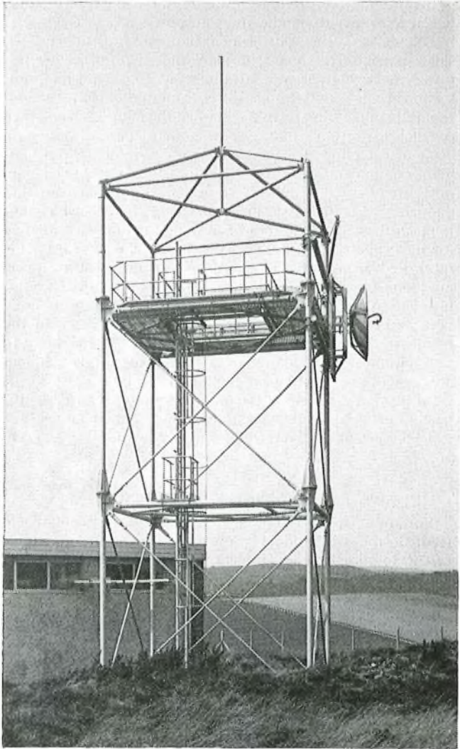
FIG. 18—A 45 ft high Tower No. 4A
