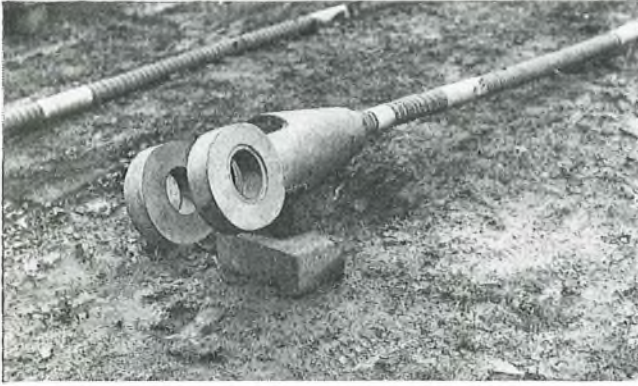
FIG. 12—Socket termination on 1\frac{3}{4} in diameter spiral-strand mast guy
