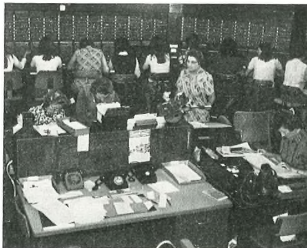
View of the Manual Exchange switch room during the last hours of its life
