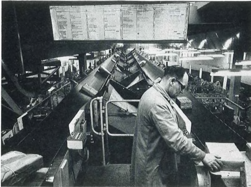
FIG 9—Tilted-belt Parcel-Sorting Machines at Worcester
