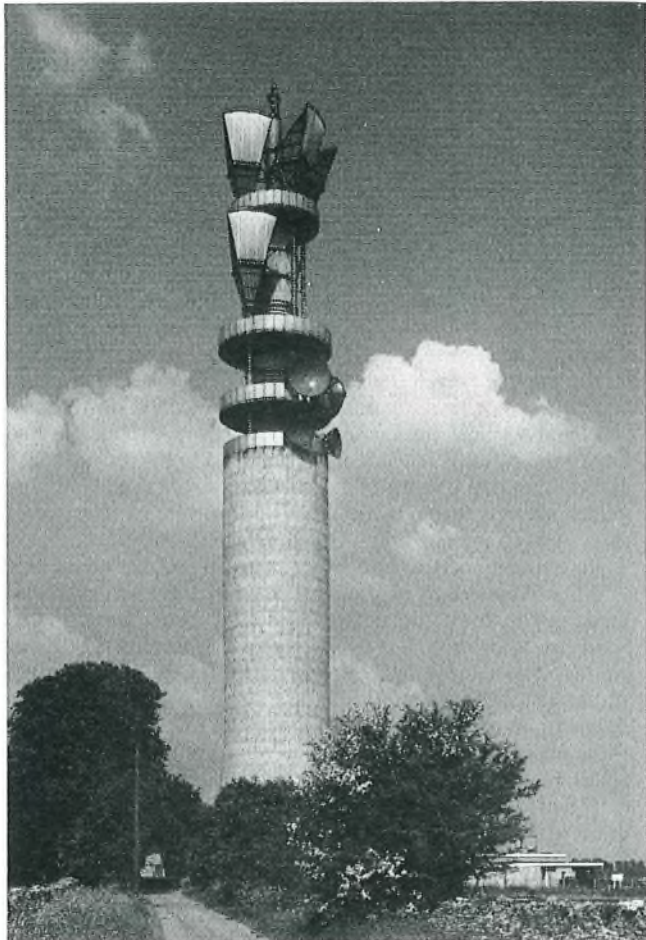
Fig. 2—An earlier type of ferro-concrete tower at Wotton-under-Edge radio station
