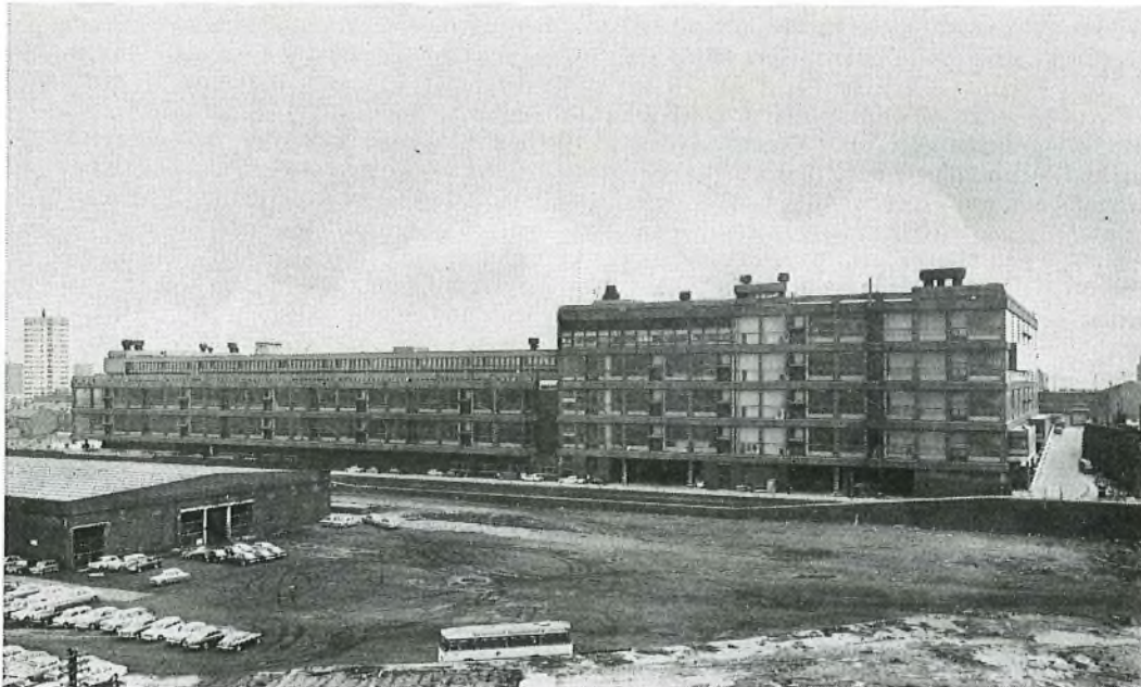
FIG. 5—The New Sorting Office at Birmingham (to be opened for service in 1970)
