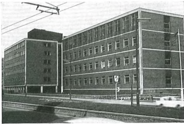
HUDDERSFIELD NEW AUTOMATIC TELEPHONE EXCHANGE
