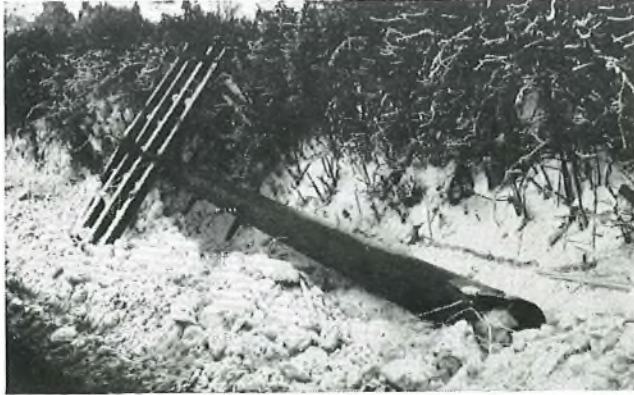
ONE OF THE COLLAPSED POLES
