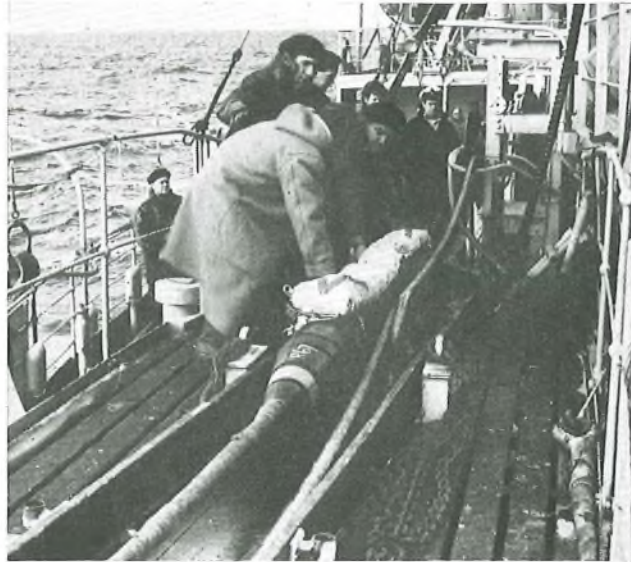
FIG. 5—LAUNCHING A REPEATER WITH PARACHUTE
