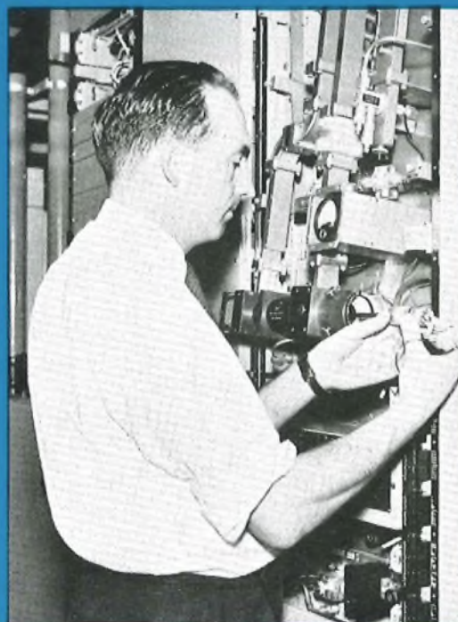
Replacing a travelling wave tube in GEC SHF radio equipment
