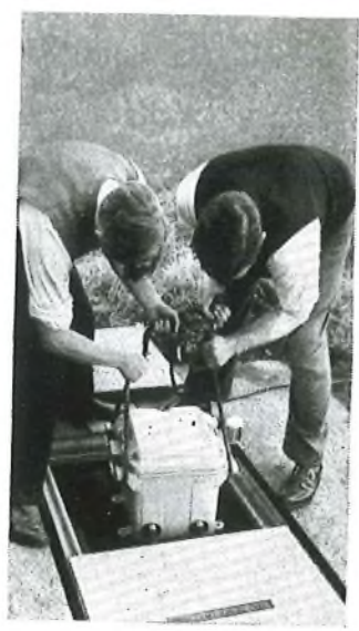
A complete 600 channel four tube repeater
