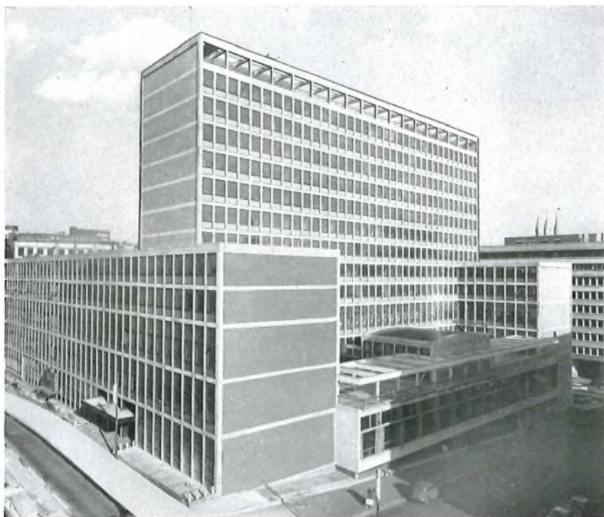
FIG. 1—FLEET BUILDING SHORTLY AFTER THE AUTOMATIC TELEX EXCHANGE WAS OPENED (10 DECEMBER 1960)
