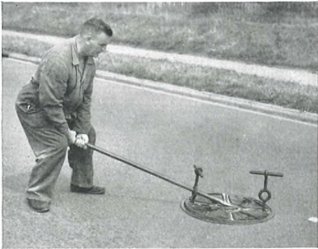
FIG. 7—EASING A MANHOLE COVER USING A CROWBAR
