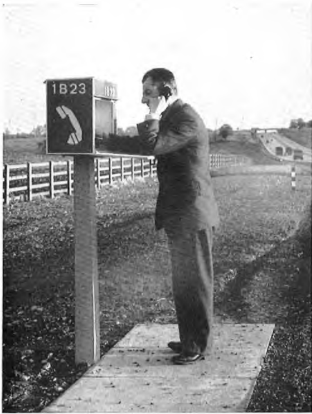
FIG. 4—GENERAL VIEW OF ROADSIDE TELEPHONE
