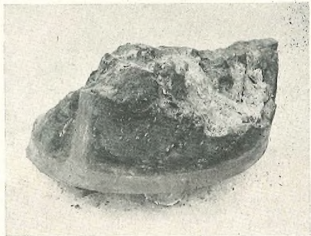
FIG. 7—PIECE OF CAST-IRON PILING AND STONY MATERIAL TREPANED FROM HARBOUR WALL
