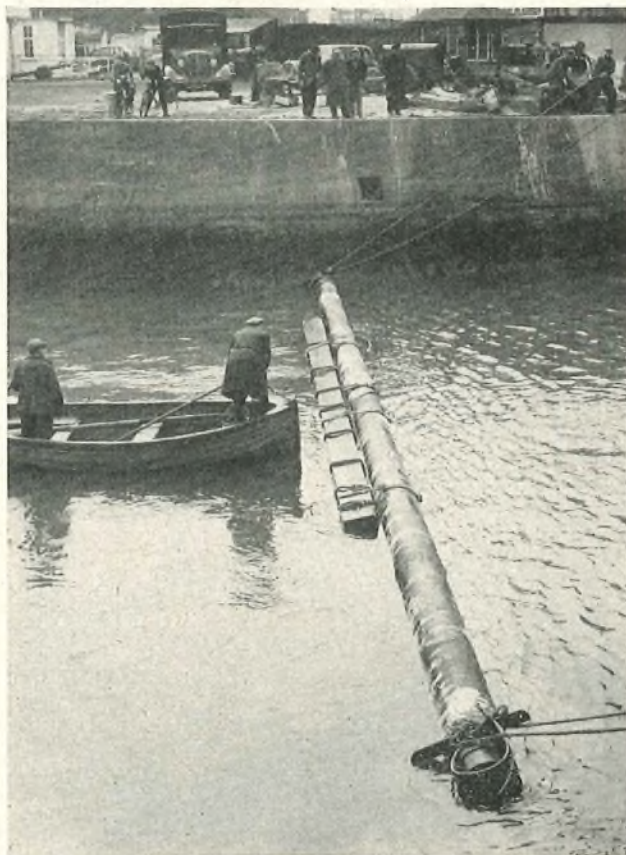
FIG. 10—MAIN-CROSSING PIPE BEING FLOATED INTO POSITION
