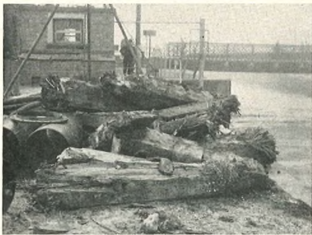
FIG. 8—OLD PILES DREDGED FROM HARBOUR BED
