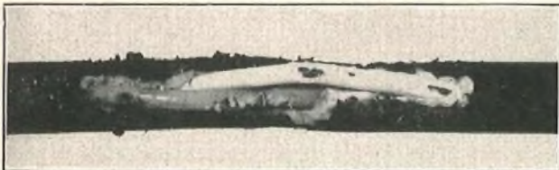
FIG. 7.—TYPICAL CASE OF DAMAGE BY VERMIN.
