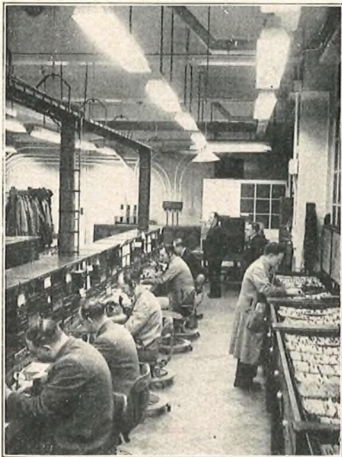
FIG. 9.—ILLUMINATION OF TEST DESKS BY FLUORESCENT LIGHTING.
