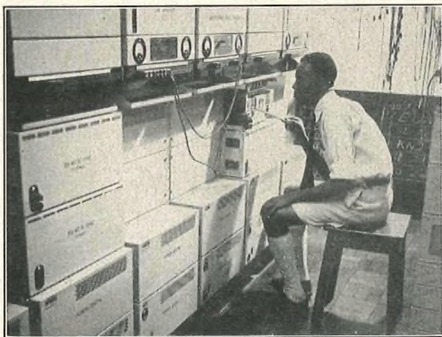
12-CHANNEL CARRIER EQUIPMENT AT KADUNA.
