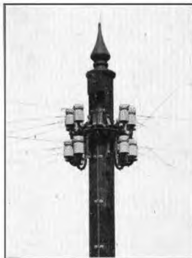
FIG. 5.—THE TOP OF A RING-TYPE DISTRIBUTION POLE.
