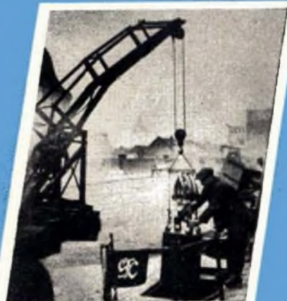
Loading coils being lowered into City street manhole
