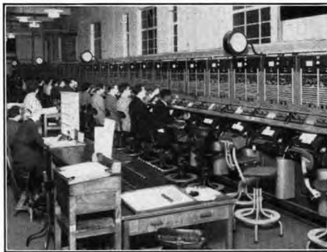
FIG. 6.—THE INTERNATIONAL TELEX SWITCHBOARD, C.T.O.
