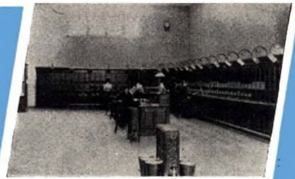
The first common-battery telephone exchange at Bristol, 1900
