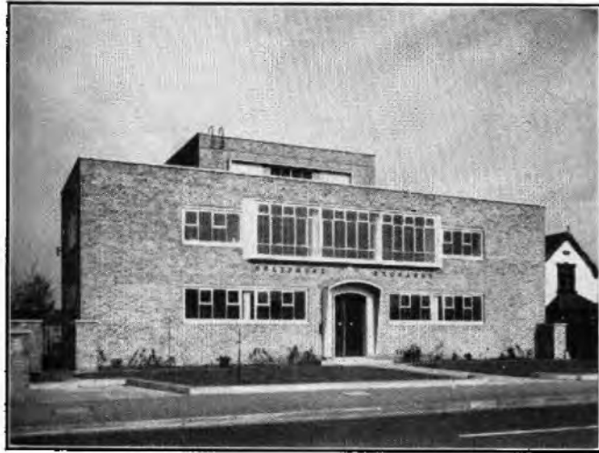
FIG. 9.—FAIRLANDS TELEPHONE EXCHANGE, SURREY.
