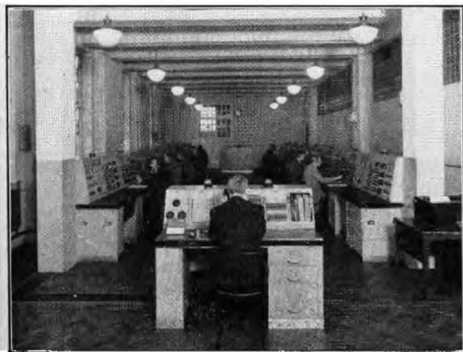
FIG. 14.—TWO SUITES OF OPERATING POSITIONS AND ASSOCIATED CONTROL POSITIONS AT THE RADIO TELEPHONY TERMINAL, BRENT.
