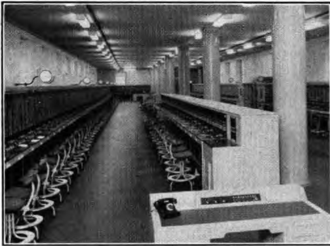
FIG. 14.—MODERN SLEEVE-CONTROL SWITCHBOARD.
