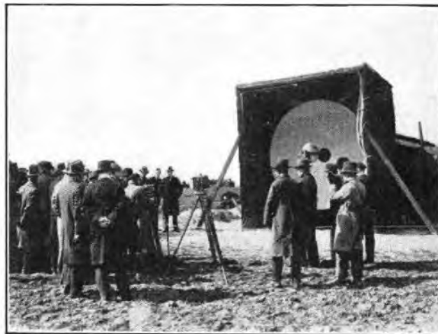
EXPERIMENTAL INSTALLATION OF MICRO-RAY SYSTEM, ST. MARGARET'S BAY, 1931.
