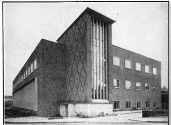
FIG. 8.—YORK TELEPHONE EXCHANGE.
