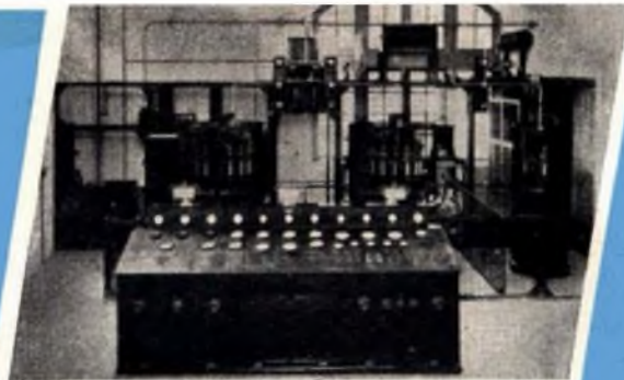
200-kW long-wave single-sideband telephony transmitter at Rugby, 1926
