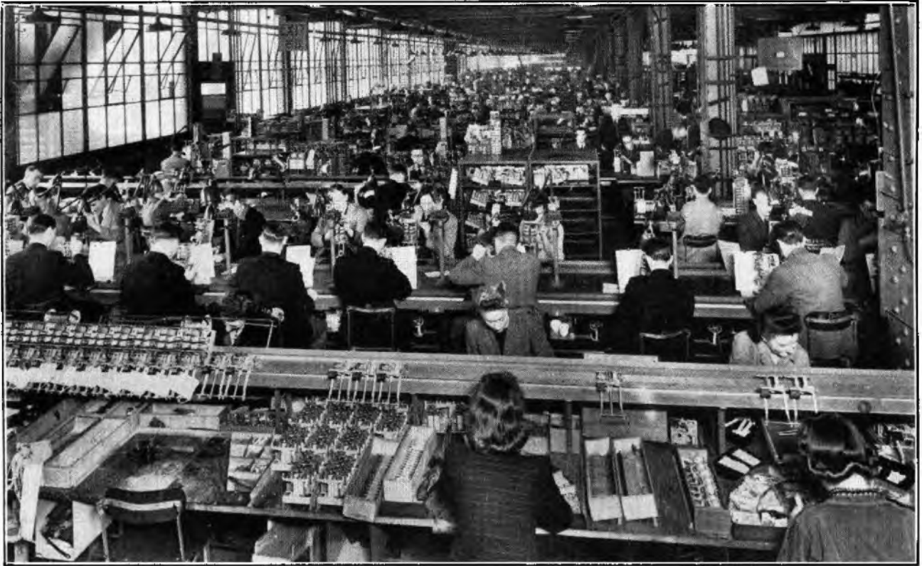
MAIN ASSEMBLY AND WIRING OF 2,000-TYPE SELECTORS.
