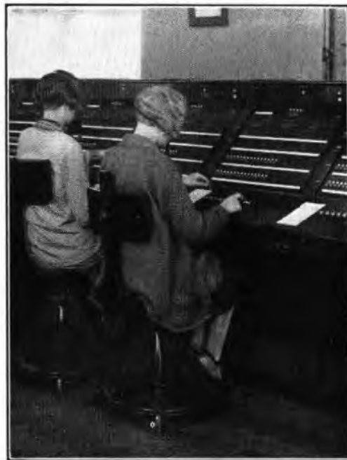
FIG. 9.—CORDLESS B POSITIONS AT A MECHANICAL TANDEM EXCHANGE.
