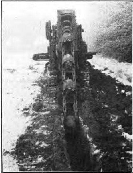
FIG. 13.—TRENCH EXCAVATOR.
