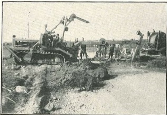
FIG. 11.—ONE OF THE TRENCHING MACHINES AT WORK.
