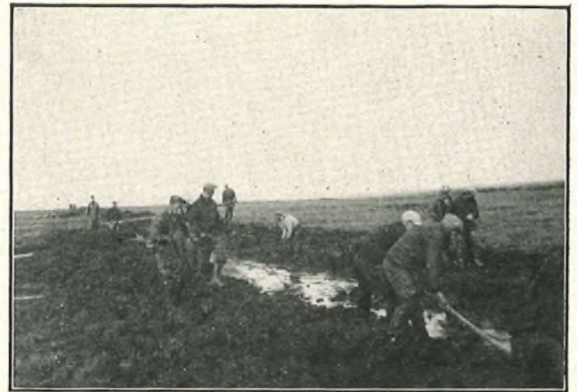
FIG. 13.—WORKING THE CABLE INTO THE TRENCH.
