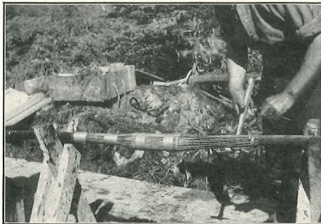
FIG. 20.—COMPLETING A SPLICE.
