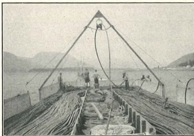
FIG. 15.—THE COILS OF CABLE ON THE DECK OF THE SCOW.
