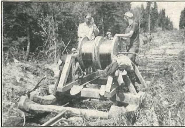
FIG. 22.—LAYING THE COPPER GUARD WIRE.
