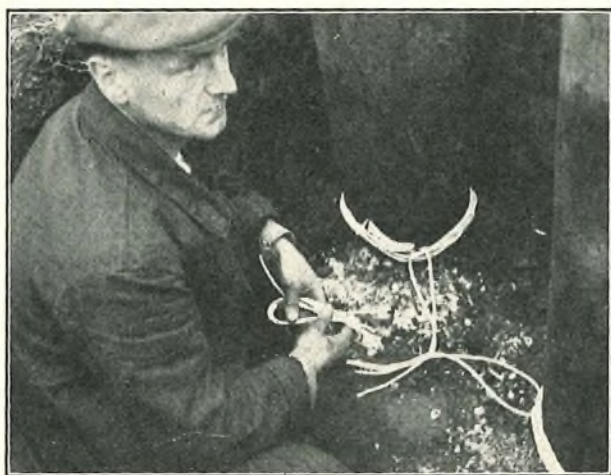
ATTACHING THE DETONATING FUSE TO A POLE.
