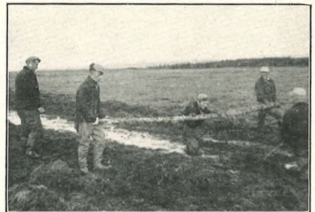
FIG. 14.—TREADING THE CABLE TO THE CORRECT DEPTH.
