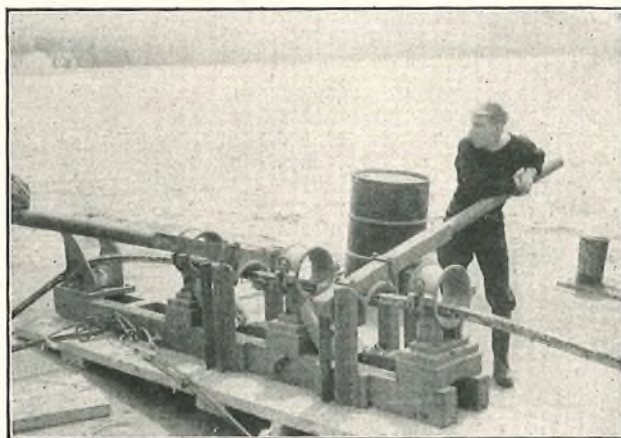
FIG. 16.—THE CABLE-BRAKING DEVICE.
