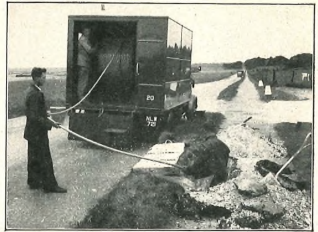
FIG. 3.—DRAWING-IN THE CABLE.
