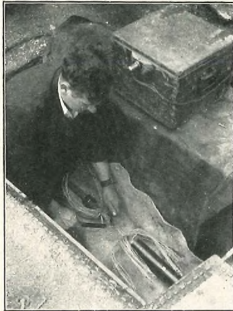
FIG. 6.—WELDING A JOINT IN THE ALUMINIUM CONDUCTORS.
