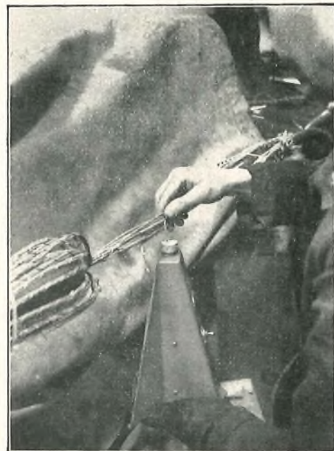
FIG. 9.—SOLDERING ALUMINIUM CONDUCTORS TO COPPER CONDUCTORS.
