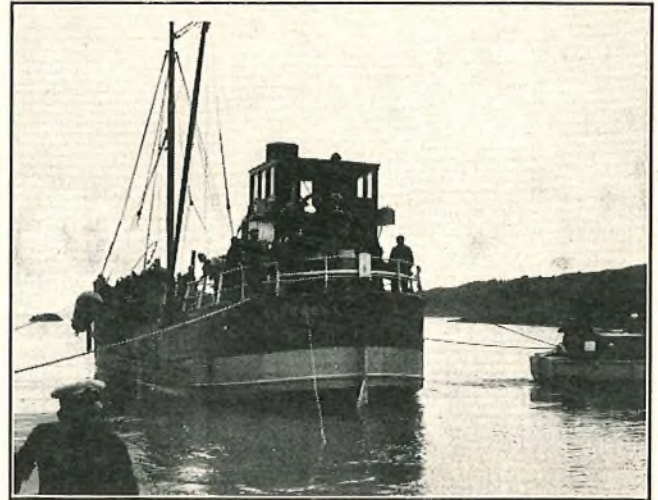
LANDING THE CABLE FROM THE "GLEN ARAY"
