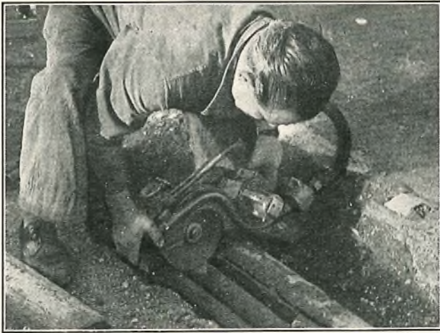
CUTTING THE STEEL PIPE.
