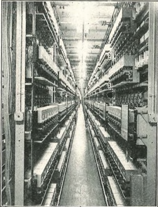
MOTOR UNISELECTOR RACKS IN KINGSWAY TRUNK EXCHANGE.
