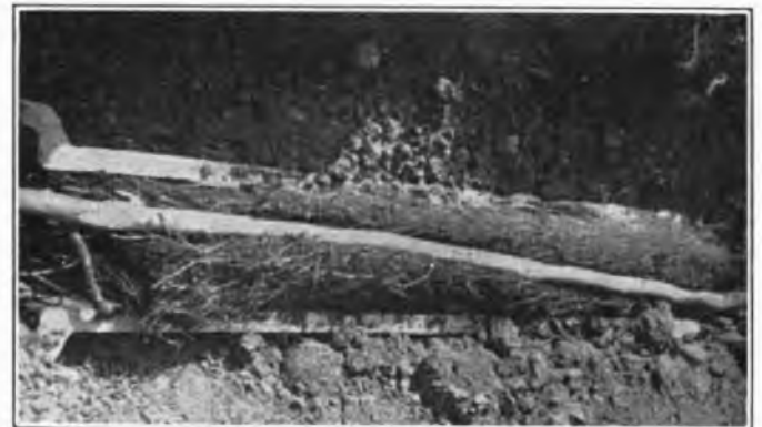
BAT WILLOW ROOTS FILLING DUCT.
