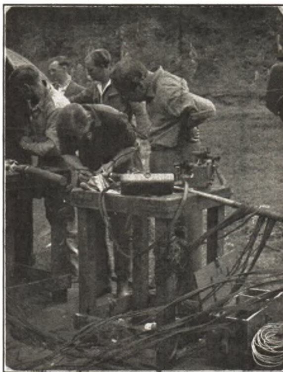
PREPARING FOR FINAL JOINTING OF LAND-SEA SECTIONS.
