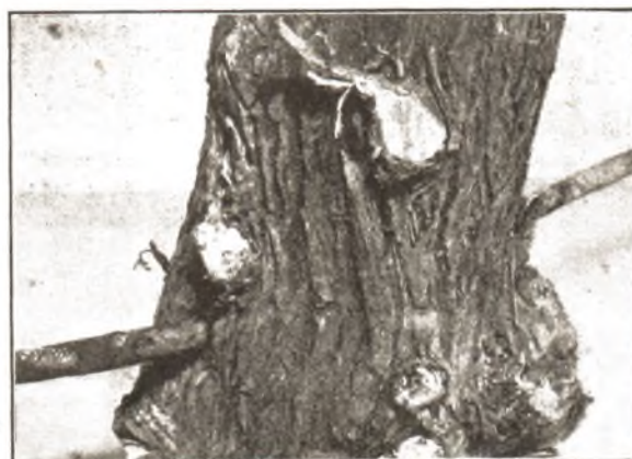
15-PR. PROTECTED CABLE EMBEDDED IN TREE.
