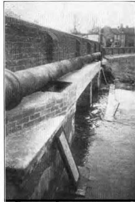
REINFORCED CONCRETE TROUGH PROVIDED ON HERMITAGE BRIDGE, EMSWORTH.
