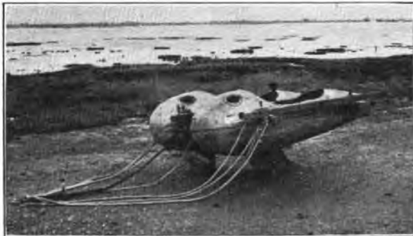
THE MOLE DRAINING RAFT, SHOWING STEERING TACKLE AND CENTRE PLATE.
