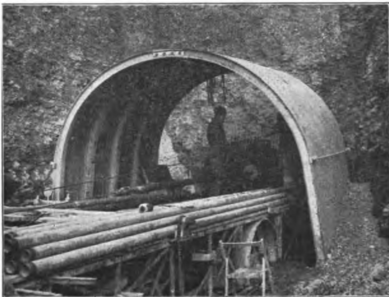
FIG. 8.—DRILLING RIG AT ENTRANCE TO LATERAL BOREHOLE.
