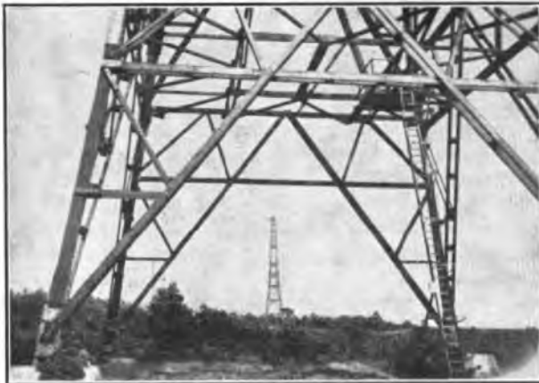
FIG. 1.—BASE OF ONE OF THE MASTS.
