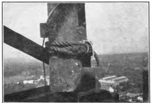
FIG. 3.—LASHING AT BUTT OF DERRICK.
