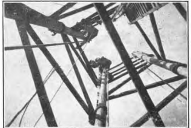
FIG. 2.—DERRICKS LASHED IN POSITION.
