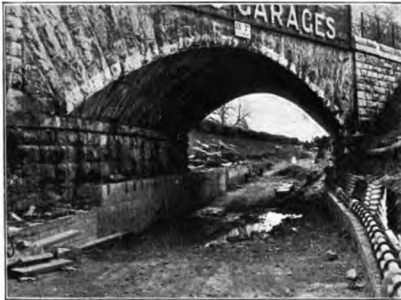
SKEW BRIDGE, SHOWING NEW POSITION OF P. O. PLANT.
