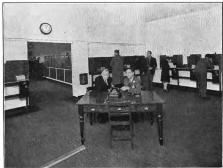
FIG. 9.—PUBLIC TELEPHONE BOOTHS IN POST OFFICE.
