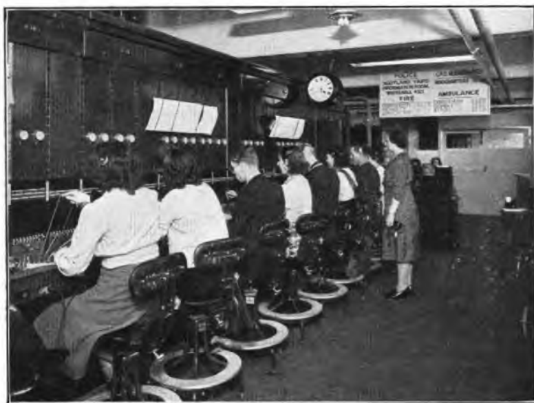
FIG. 1.—CORINTHIAN EXCHANGE—PART OF SWITCHBOARD
