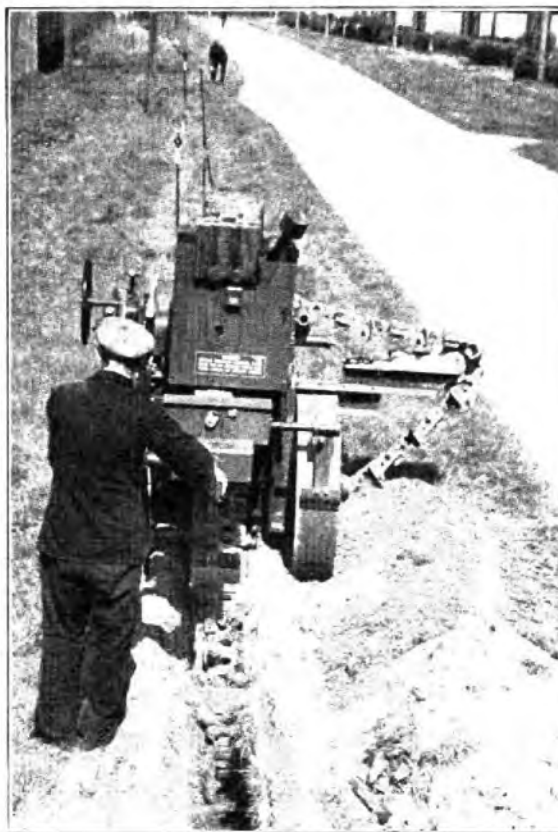
FIG. 2.—CUTTING A TRENCH.
