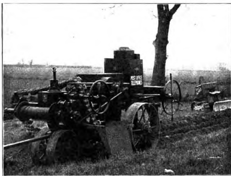
FIG. 1.—AVELING-BARFORD TRENCH-CUTTING MACHINE.
