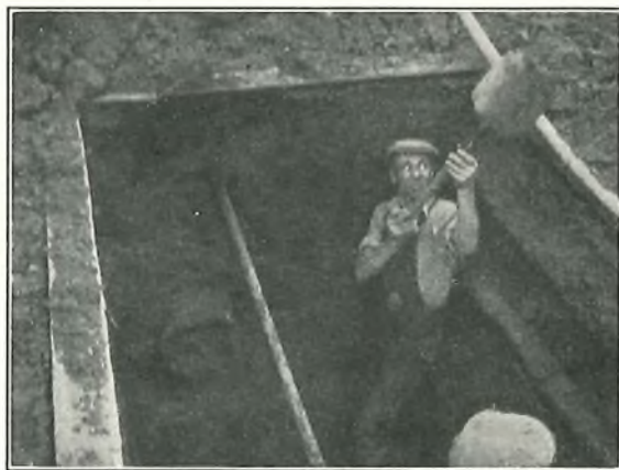
FIG. 5.—MANHOLE EXCAVATION IN WET SITUATION.
